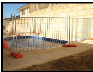
Temporary pool fencing during pool construction
